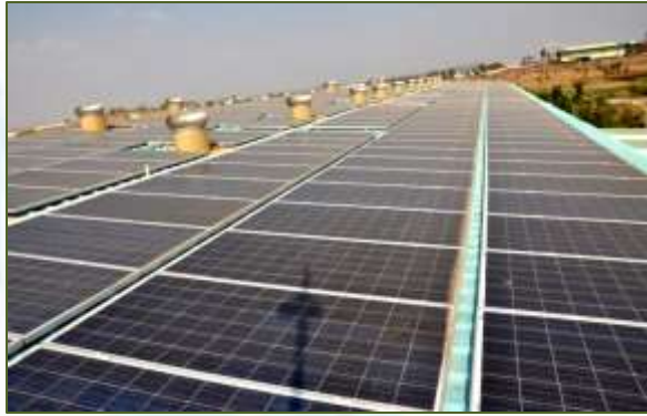
Use of renewable source of energy (Solar Power)
