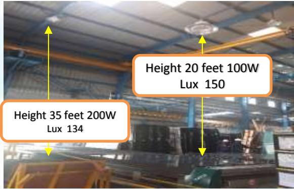
Reduction in Induction Lamps height on shop floor
