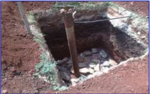
Tank overflow water to Rain water harvesting pit
