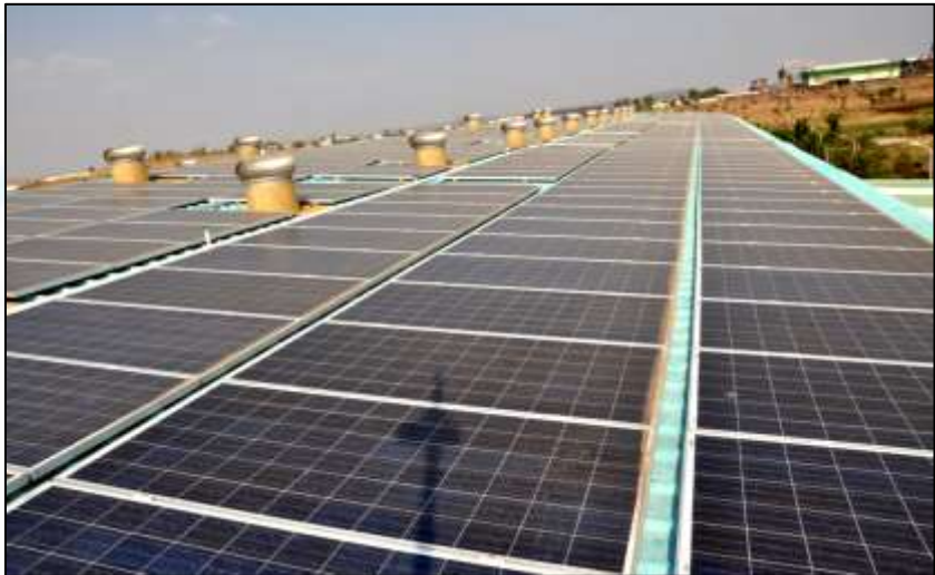
Solar Power Generating electricity 3,28,500 kWh / Year
