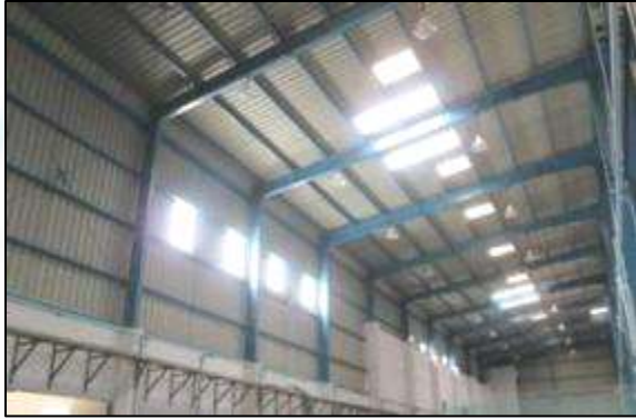
Transparent sheets for roofing at regular intervals
