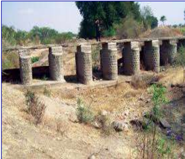
Construction of "Bund" at village - Salav for collecting rainwater (Capacity – 12 Lacs Litre)
