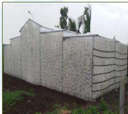
Green House from recyclable & waste material
